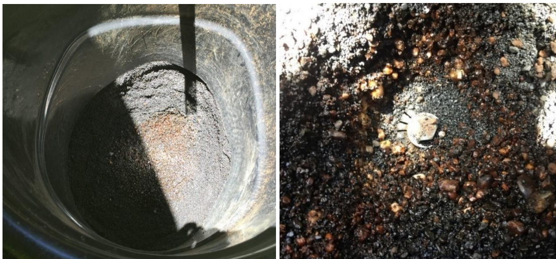
Figure 3-5: Filter nozzle exposed with coal with gravel and media intermixing
